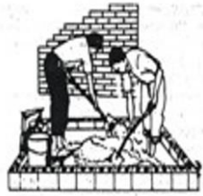
Plate 1: Men mixing concrete with spade
